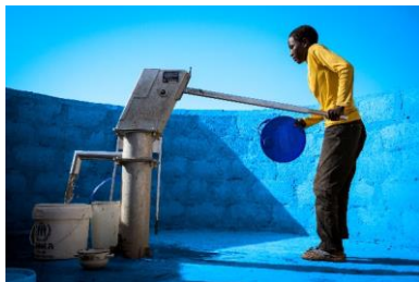
Handpump borehole
